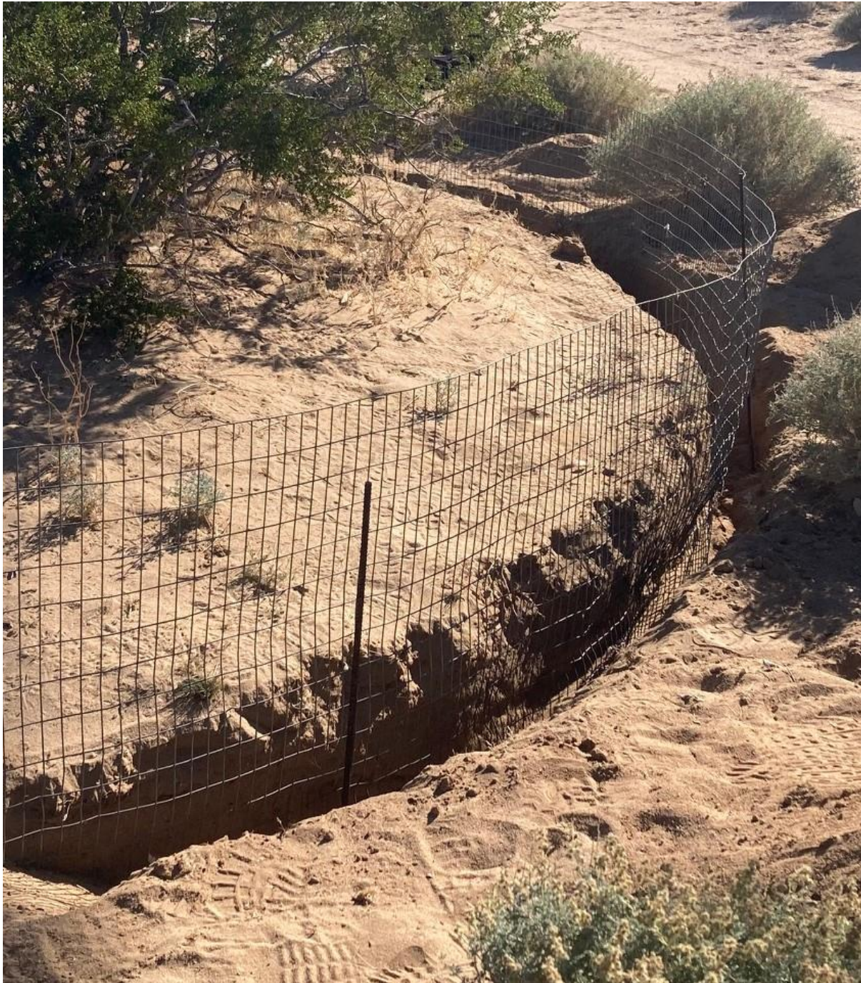
Figure 6. Example of fencing designed for the temporary penning of a desert tortoise. Note: this fencing is currently under installation; the open trench at the base of the fence must be backfilled to eliminate gaps that could entrap tortoises.
